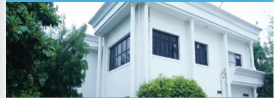
State-of-the-art D9 US FDA accredited API facility at Panoli, Gujarat
