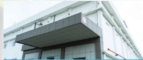
State-of-the-art T20 US FDA accredited solid dosage manufacturing facility at Panoli, Gujarat
