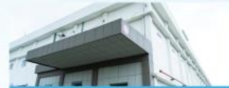
State-of-the-art T20 US FDA accredited solid dosage manufacturing facility at Panoli, Gujarat
