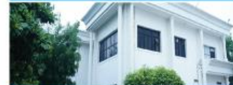
State-of-the-art D9 US FDA accredited API facility at Panoli, Gujarat
