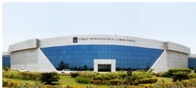
State-of-the-art Formulations manufacturing facility at Panoli, Gujarat
