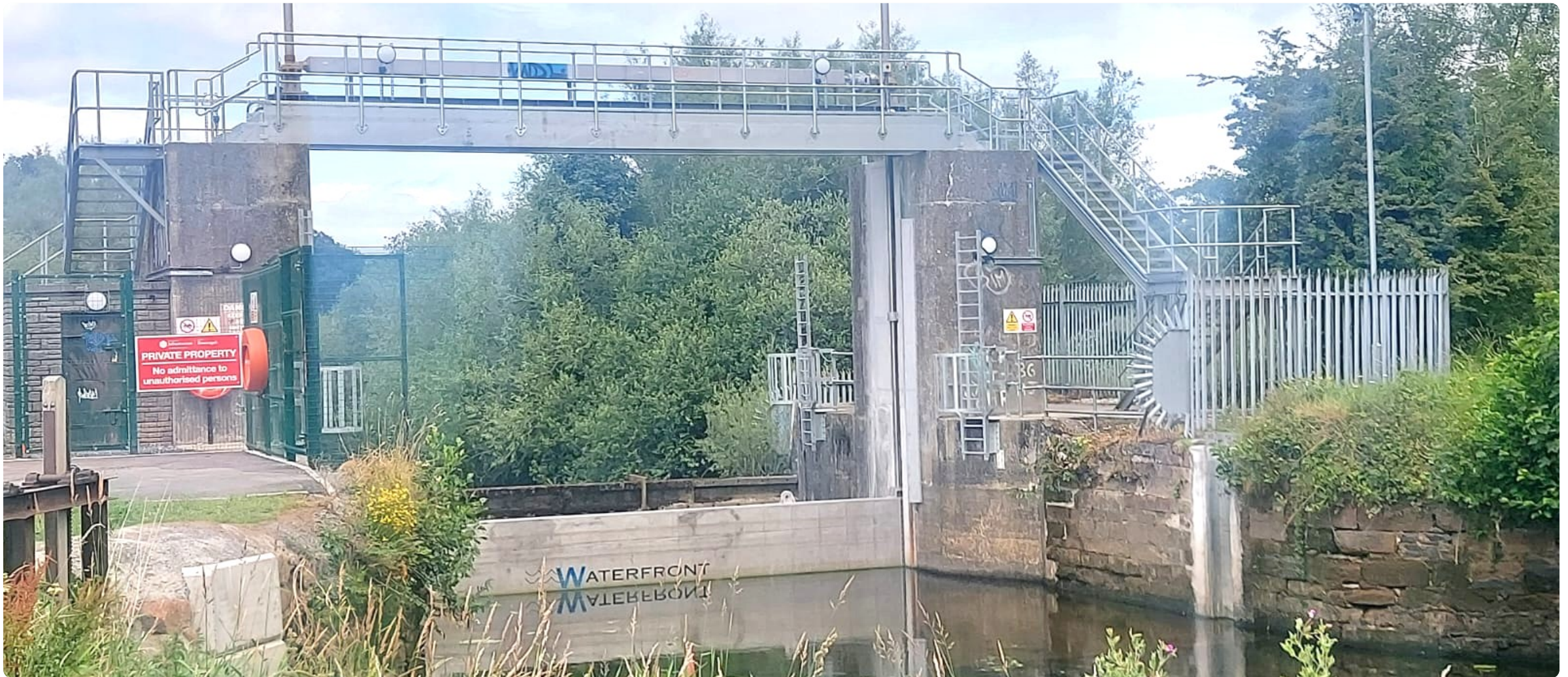
Roller Gate, Size: 10040 mm (W) X 2000 mm (H)
