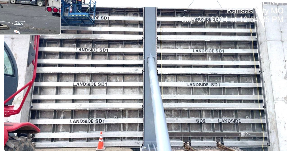
Aluminium stoplogs, Size – 23' X 4' and Structural steel stoplogs, Size – 40' X 2'
