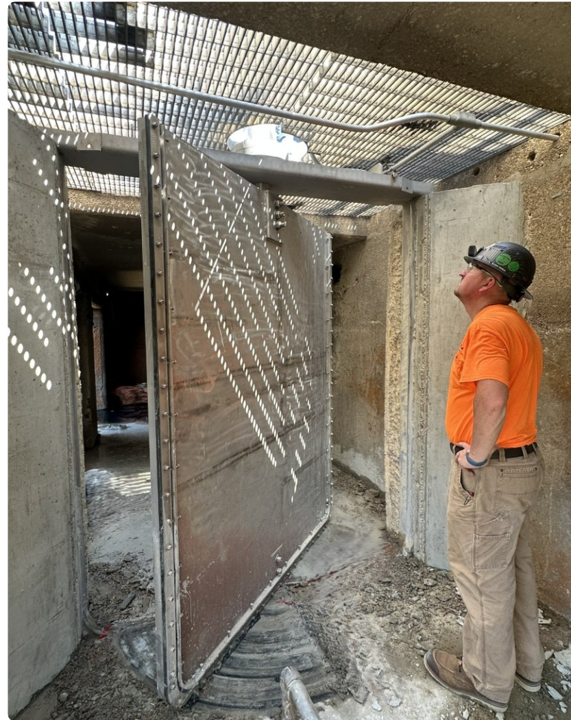
Stainless steel butterfly gates, 6' (1830 mm) X 5' (1525 mm) – 6 Nos.
