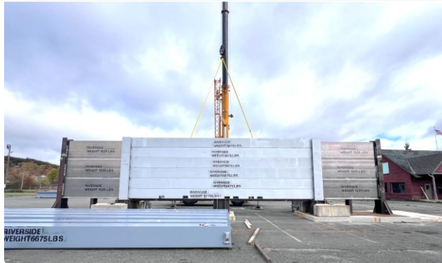
Aluminium stoplogs, Size – 23' X 4' and Structural steel stoplogs, Size – 40' X 2'
