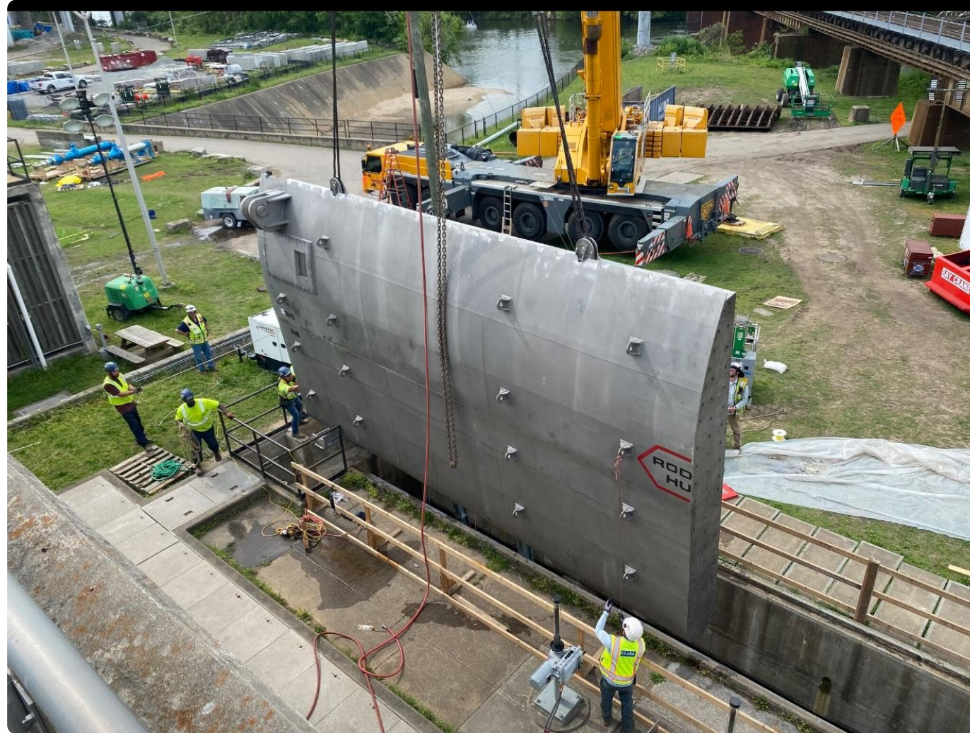
Stainless Steel Crest Gates, Size: 54' x 12' (16.5 x 3.7 m)
