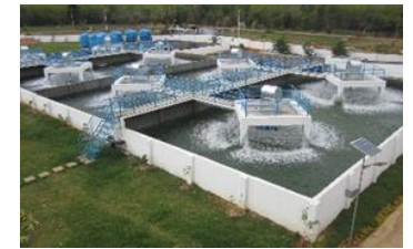
Slow speed fixed aerator
