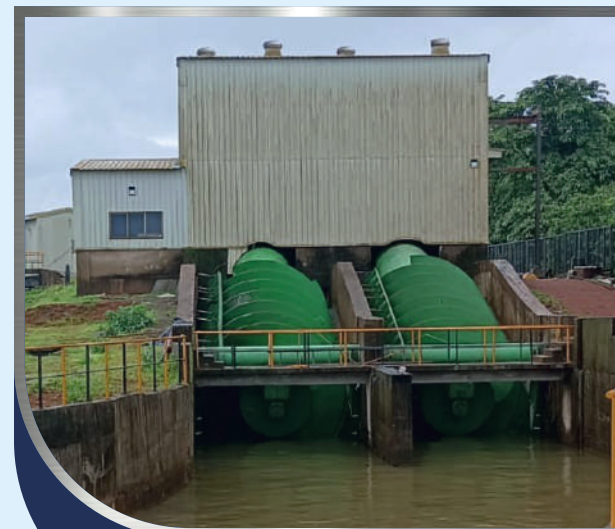
Tillari Left Bank Canal, Bhedshi, Maharashtra
