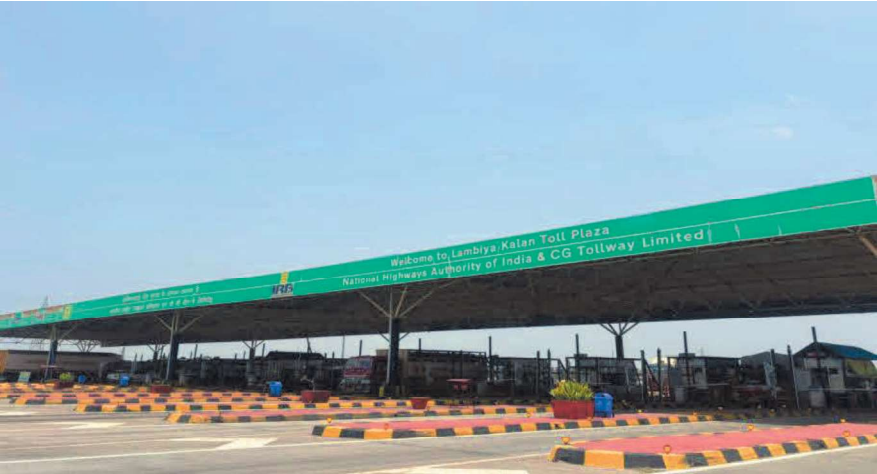
Appendix 2 (b): Site Visit - CGTL – Lambiyan Kalan Toll Plaza
