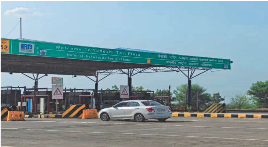
Appendix 2 (c): Site Visit - SYTL – Yedeshi Toll Plaza
