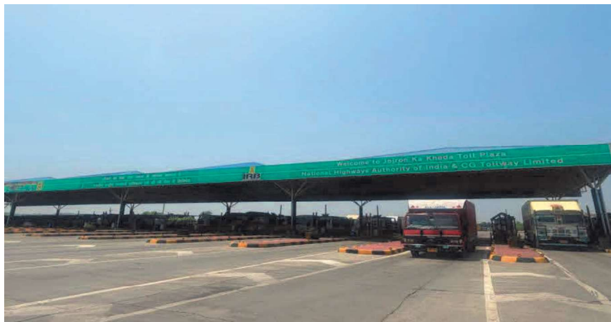
Appendix 2 (a): Site Visit - CGTL – Jojaro Ka Kheda Toll Plaza
