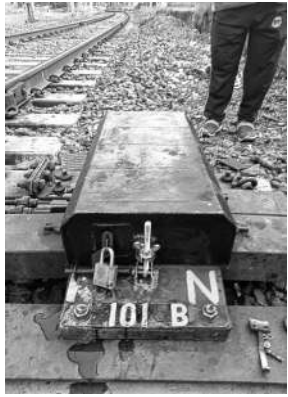
New covers keep the point machines dry
