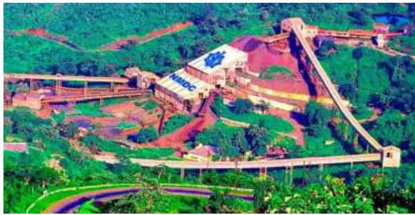
CAPEX PLAN. Nearly ₹12,000 crore worth of expansion projects are underway and expected to be completed over the next three years
