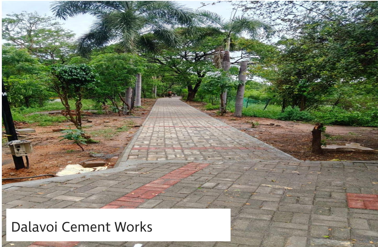
Lake Pathway and Renovation Work In Dalavoi Tamilnadu
