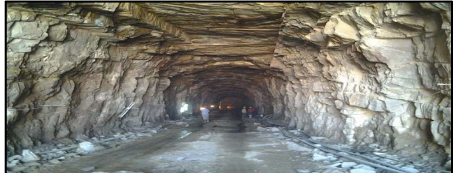
Pranahita - Adit Tunnel-Hard Rock Excavation Completed Stretch
