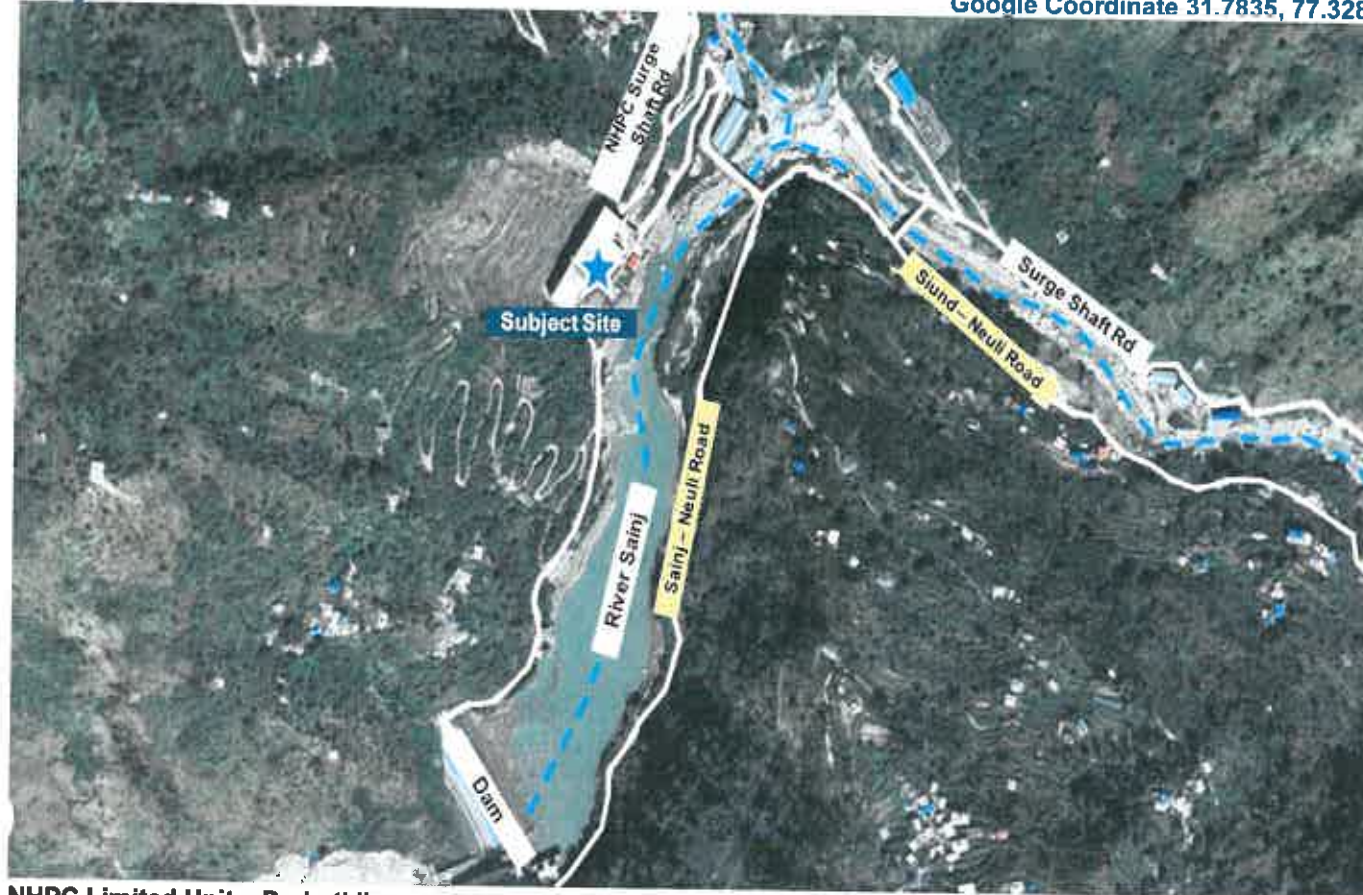
NHPC Limited Unit – Parbati II
