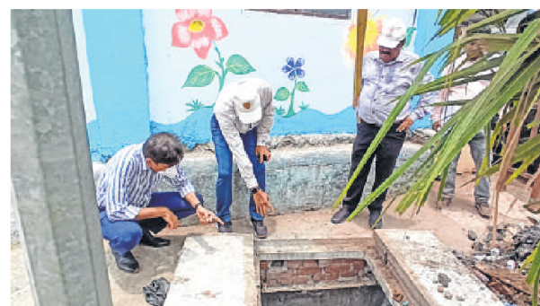
NMMC chief Abhijit Bangar (left) along with civic officials inspecting a site on Friday
