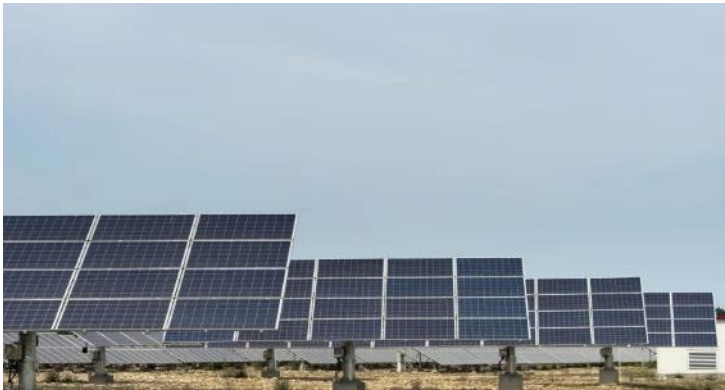
First fully integrated Energy Management System (EMS) deployment at a renewable energy facility
