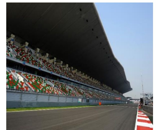
Grandstand Roofing at Buddh Int'l Circuit
