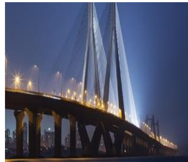
Toll Plaza at Bandra-Worli Sea Link
