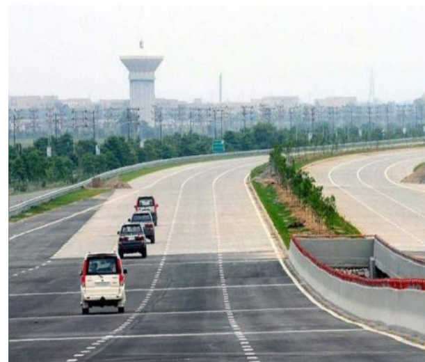
Crash Barrier at Yamuna Expressway
