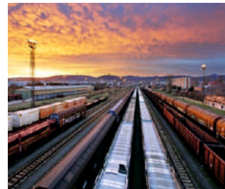
Dedicated Freight Corridor
