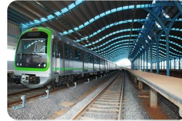
Railway Infrastructure & Airport
