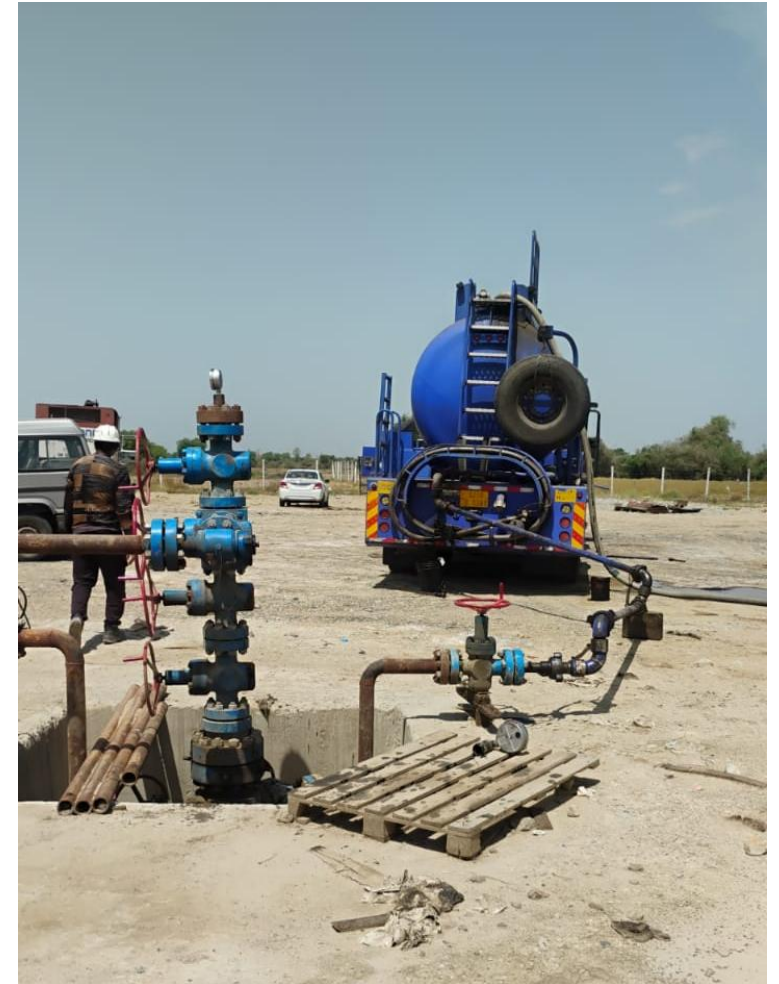
Hot water circulation job carried out in NB-11
