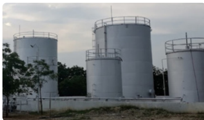
Fig. 5: Green Oil is stored on-site, where Carbon Slurry is separated
