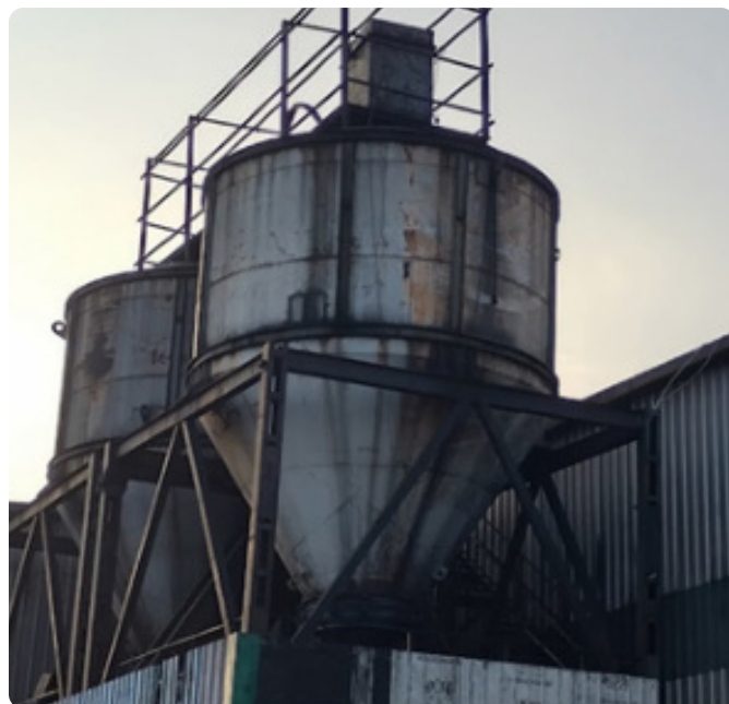
Fig. 7: Storage for rCB, used when kiln is shut down for cleaning
