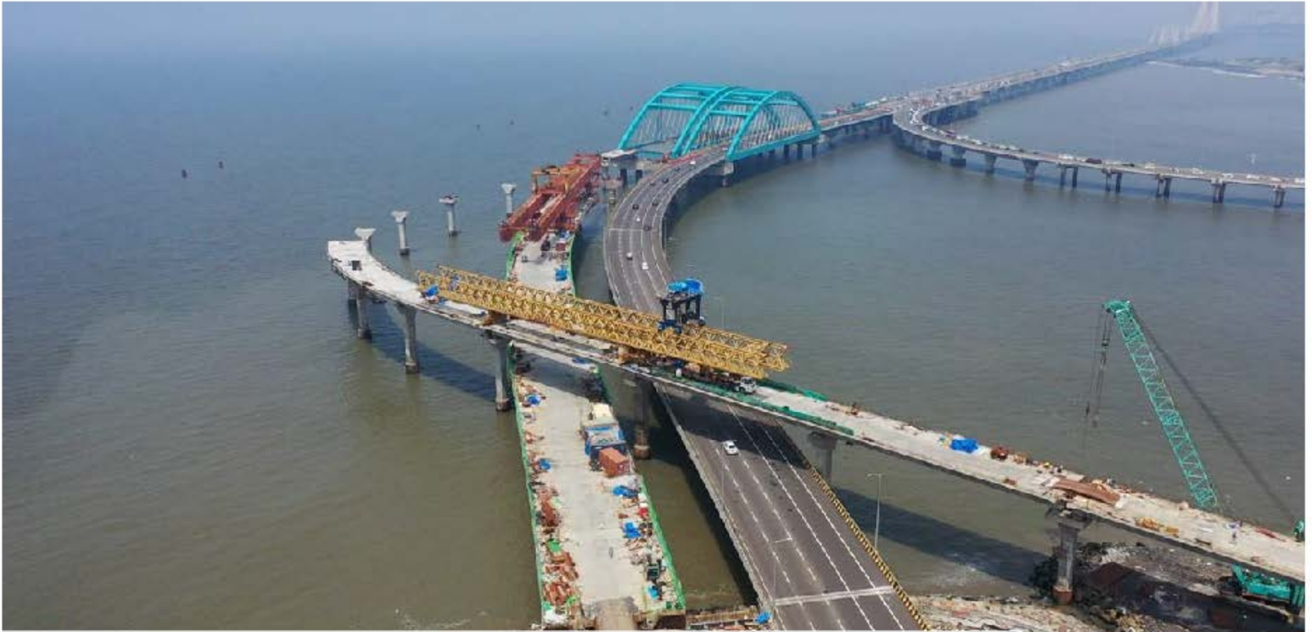
Main Bridge Segment Launching works
