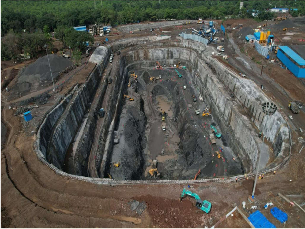
Powerhouse Excavation
