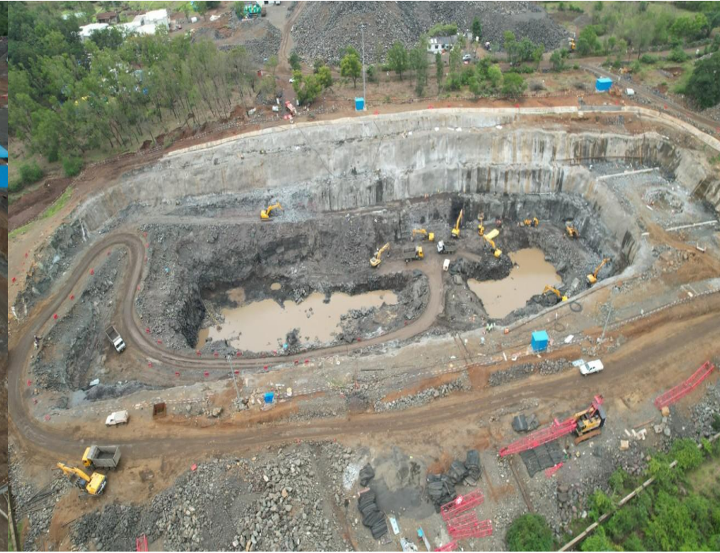
Upper Intake Excavation
