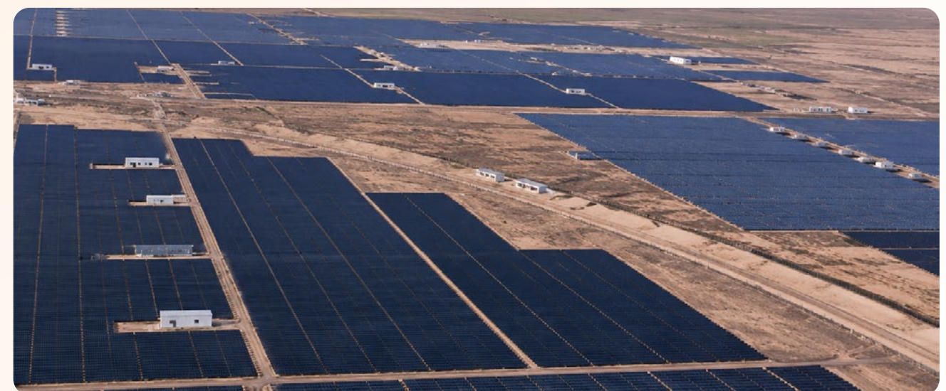
75 MW Group-Captive Solar Power Project
