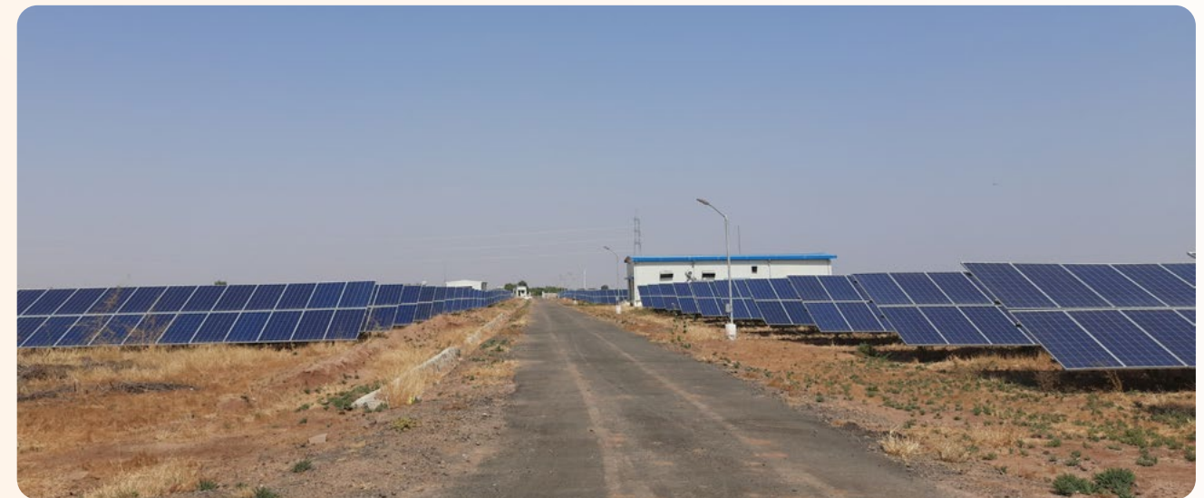
15 MW Charanka Solar Power Project
