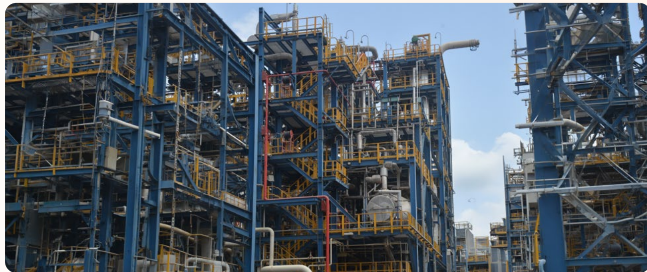
Urea-II Revamping Project
