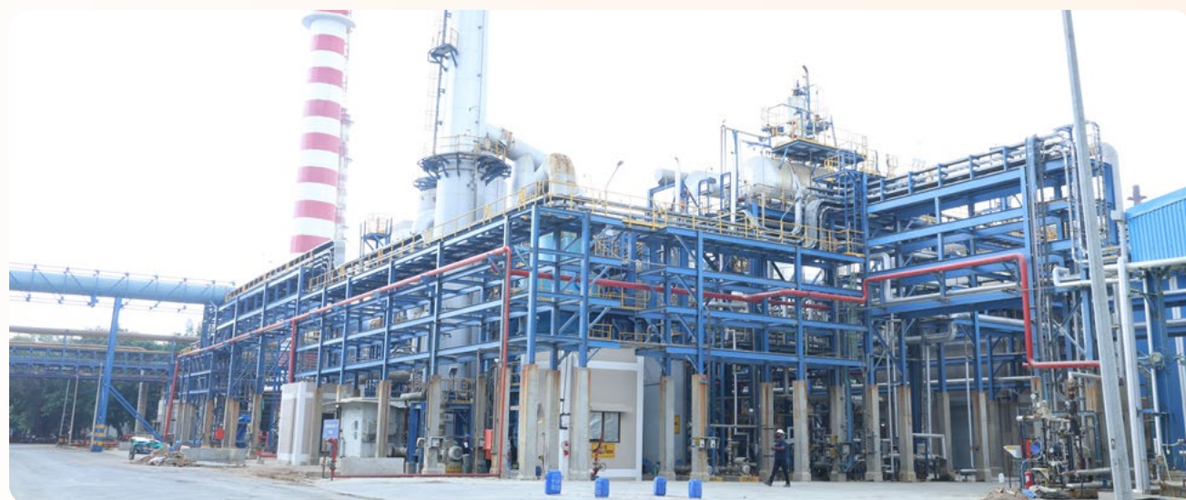
600 MTPD Sulphuric Acid-V Plant
