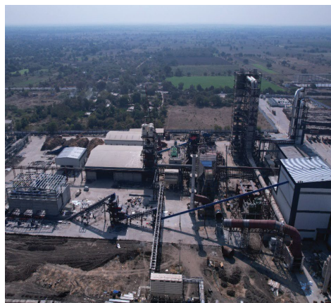
Greenfield MDF Board Manufacturing Facility at Vadodra, Gujarat
