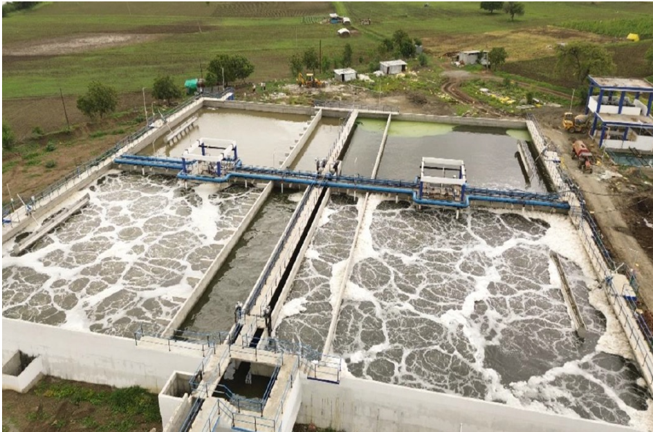
32 MLD STP Plant at Latur, Maharashtra
