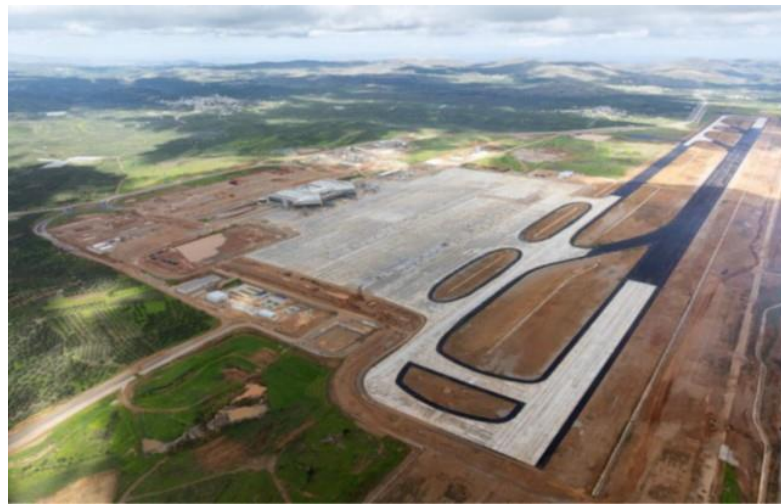
Airside Pavement Works
