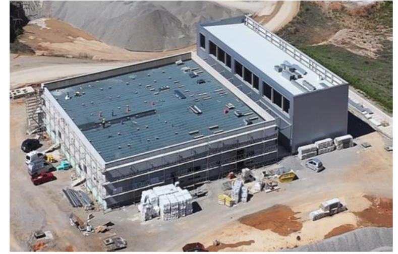
Power Plant Building
