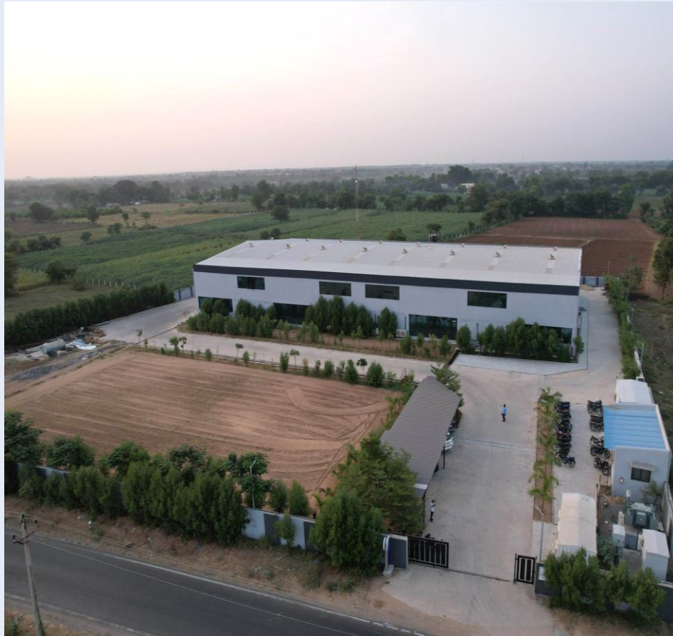
Survey No. -319 Old Block Survey No. 319, 320, 321 Industrial factory Building at Mouje, Tundali, Mahesana, Gujrat
