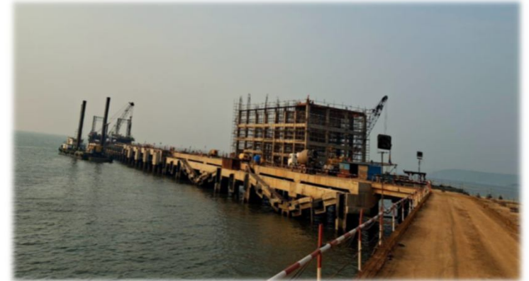
LPG construction at Jaigarh Port
