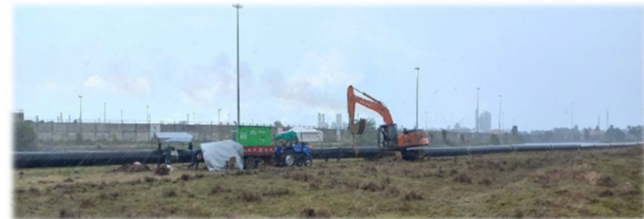
Setting up slurry pipeline
