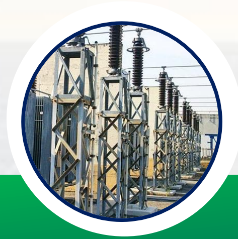
Installations of Electrical Sub Stations
