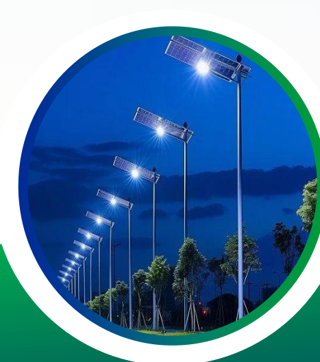
Solar Street Lighting System
