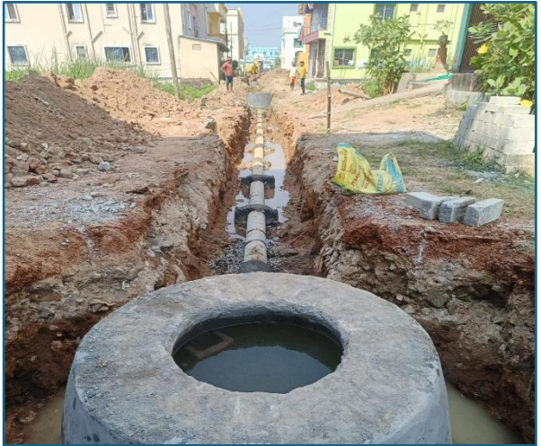
Hydrotest Checking at Lingipur
