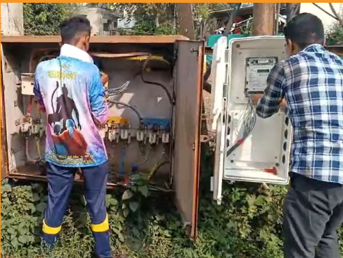
Successfully installed digital smart meters across Maharashtra for Adani Energy: our expertise in large-scale utility Infra
