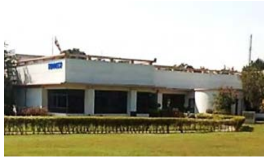
Chakan Sealings Facility (FMSIL)
