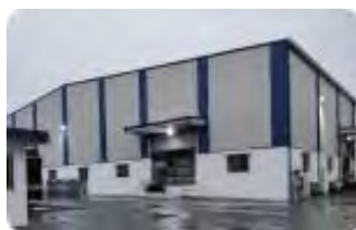
Chakan ART Facility
