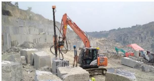
Excavator-mounted Mechanical Drill
