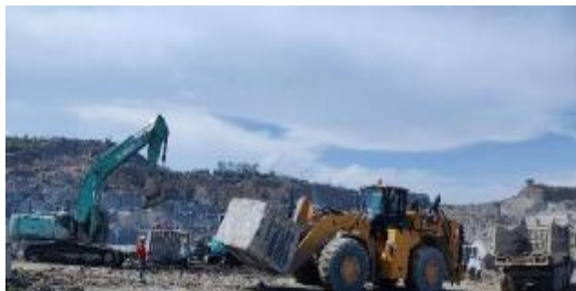
Wheel Loader with Excavator in foreground
