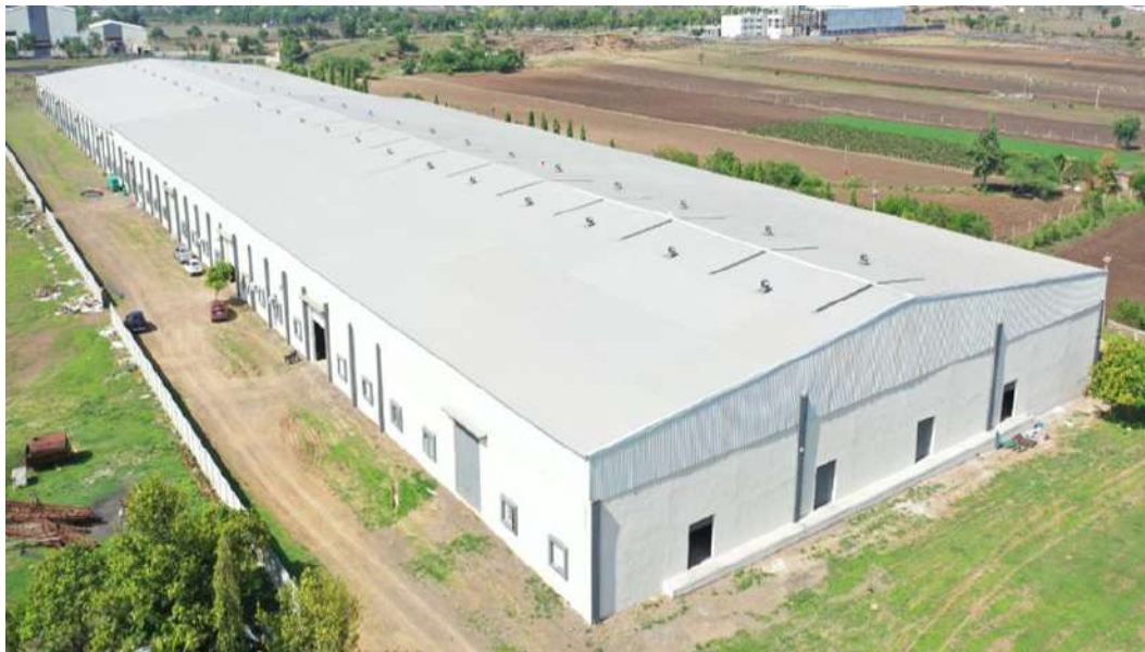
(Padavala / Existing Facility 3)
