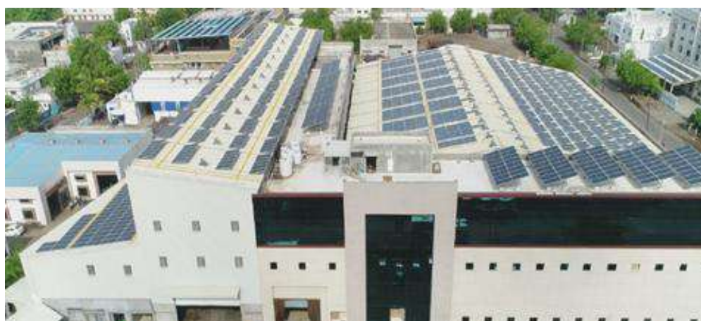
(Metoda / Existing Facility 1)
