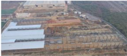
Phase II (Under Construction)
