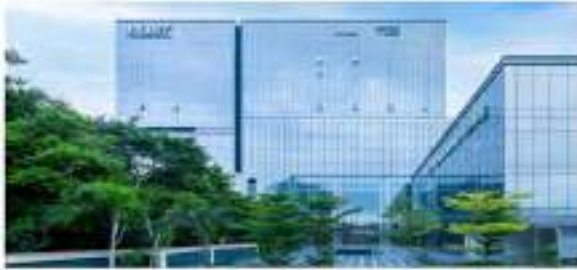
WeWork HQ27, Gurgaon
