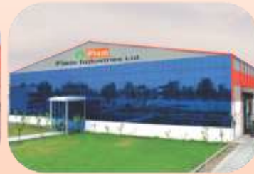
Unit-9, Ahmedabad (Gujarat)
