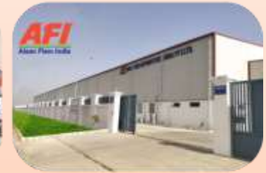
Unit-10, Tapukara (Rajasthan) Aisan Fiem Automotives India Pvt. Ltd.
