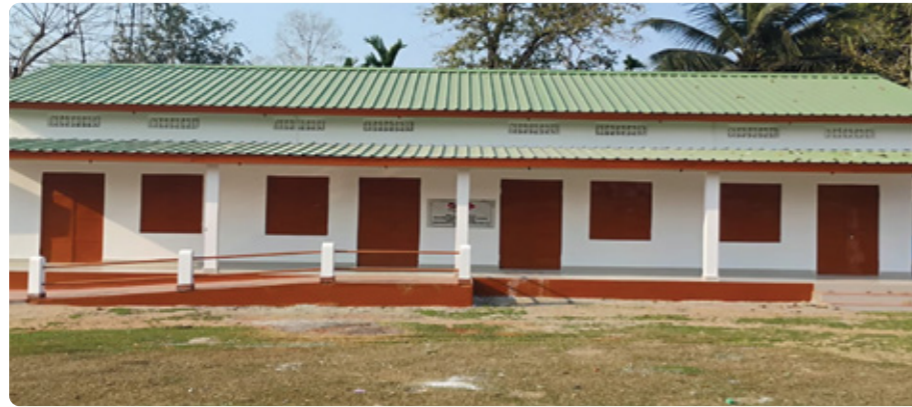
Infrastructure upgradation of Dalgoma Higher Secondary School, a co-educational government institution in Matia, Goalpara district, Assam.
