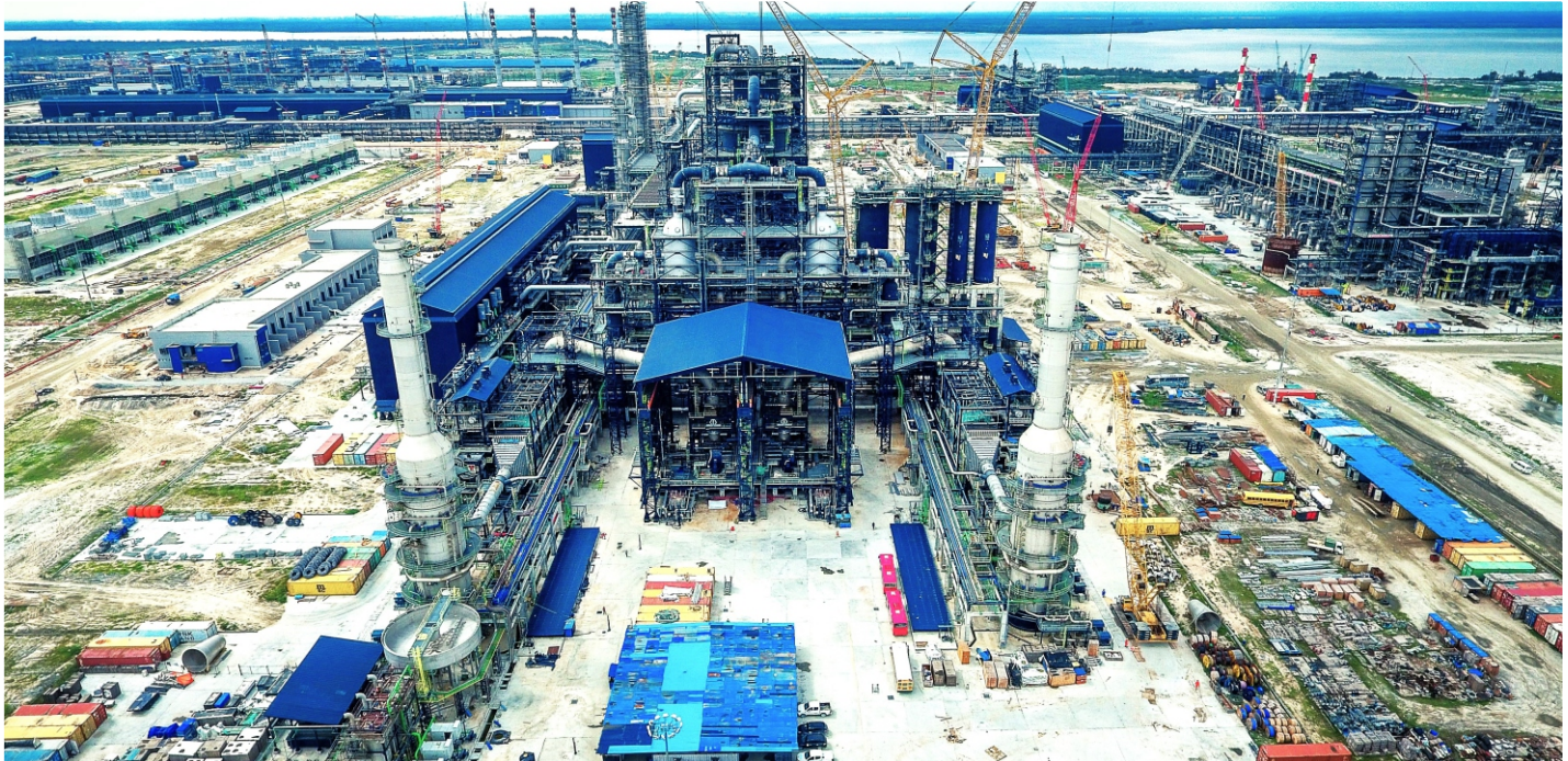
Dangote Refinery Project, Nigeria
