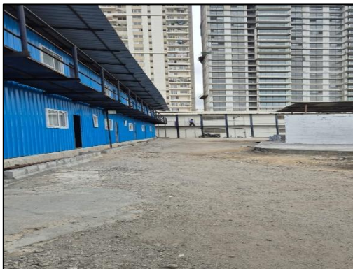
View of the Subject Property (Sy. No. 58/1)
