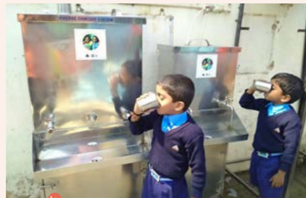
Reverse Osmosis (RO) Drinking Water Units
