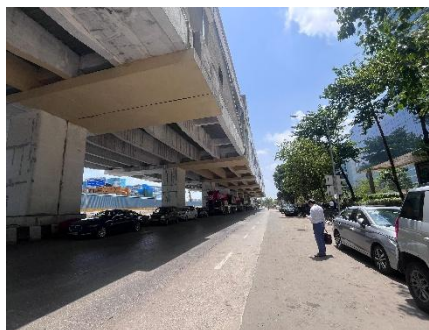
View of Access Road
