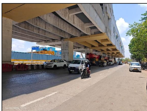
View of the Primary Access Road (Bandra Kurla Complex Road)
