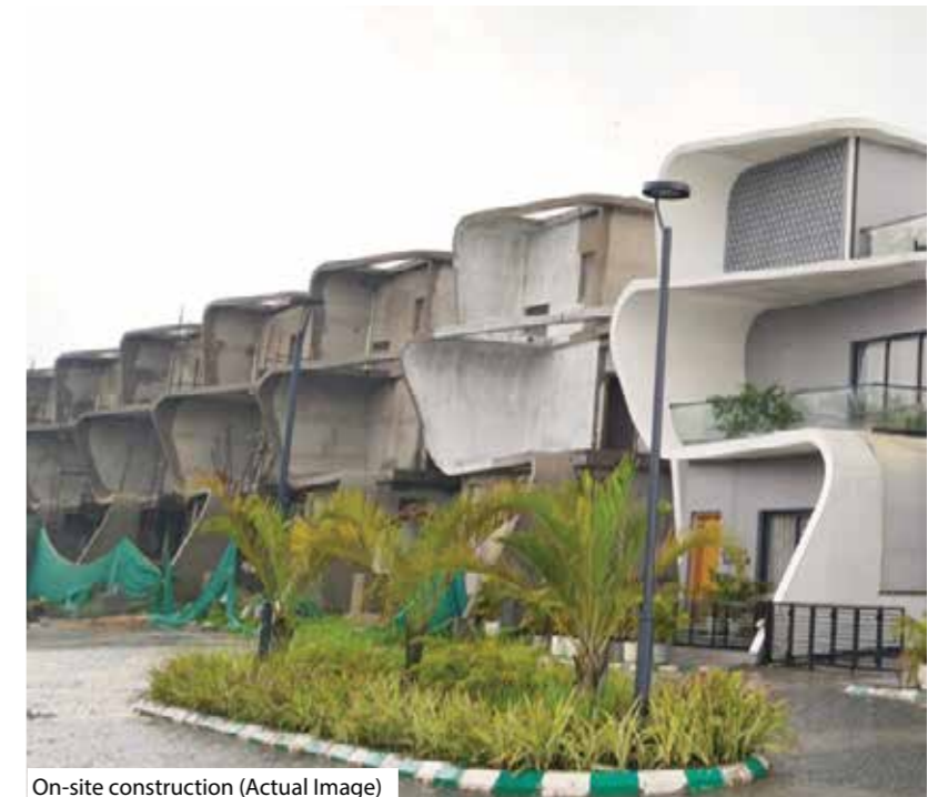
On-site construction (Actual Image)
