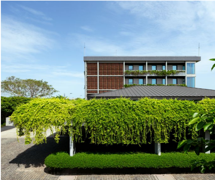
Indian Green Building Certification (IGBC) With Platinum Rating for REHQ
