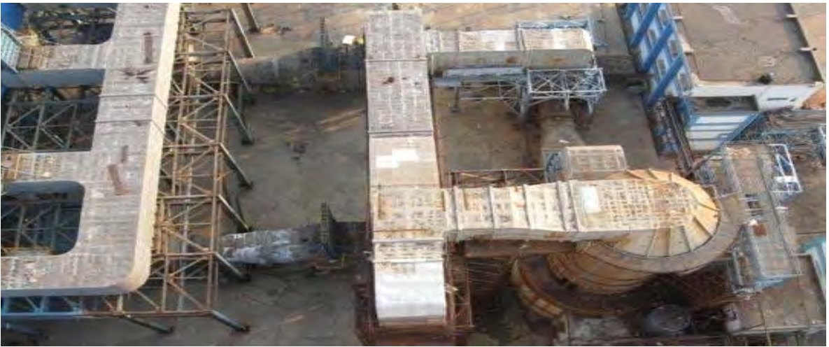
(India's first wet limestone FGD system on a coal-fired power plant with production of saleable gypsum for 2 x 600 MW Udipi Thermal Power Station, Karnataka, India, installed by our Company.)
