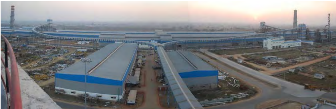
(India's Largest Material Handling system in an Aluminium Smelter at Sambhalpur, Orissa, India, installed by Our Company)
