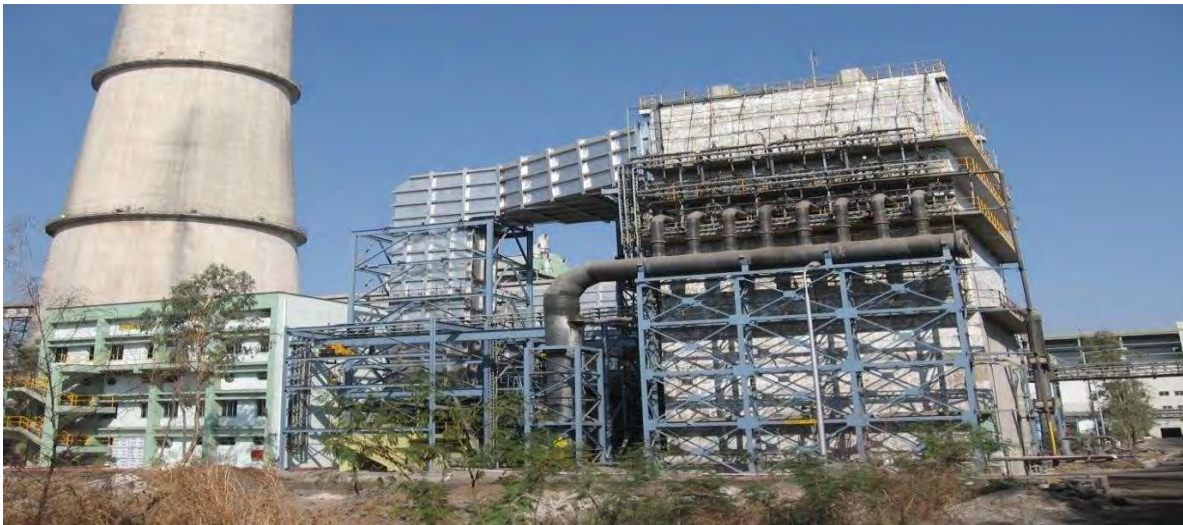
(India's first sea water FGD system with 100% of flue gas for 2 x 250 MW Dahanu Thermal Power Station at Dahanu, Maharashtra, India, installed by our Company.)
