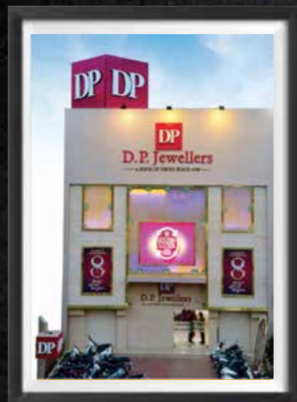
SHOWROOM AT UDAIPUR
