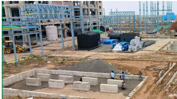
Foundation Works Completed of Isobutylene (RM) Tank
