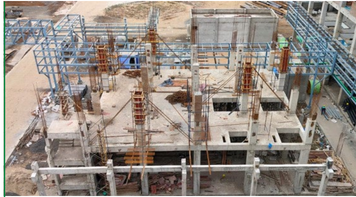
Civil Works at Recovery Plant
