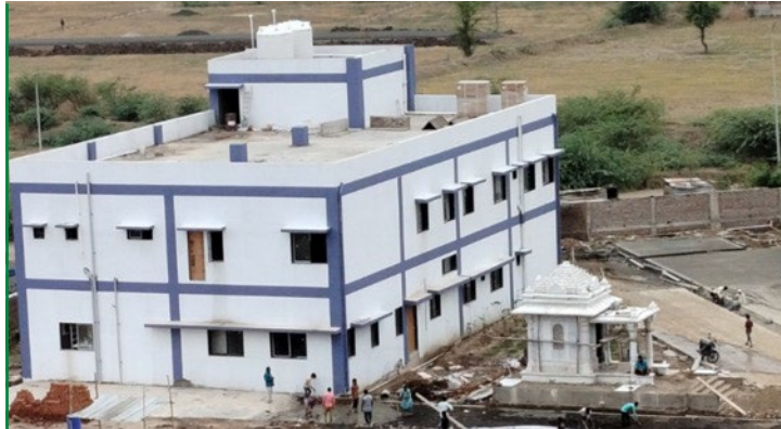
R&D and Administration Block Started in July
