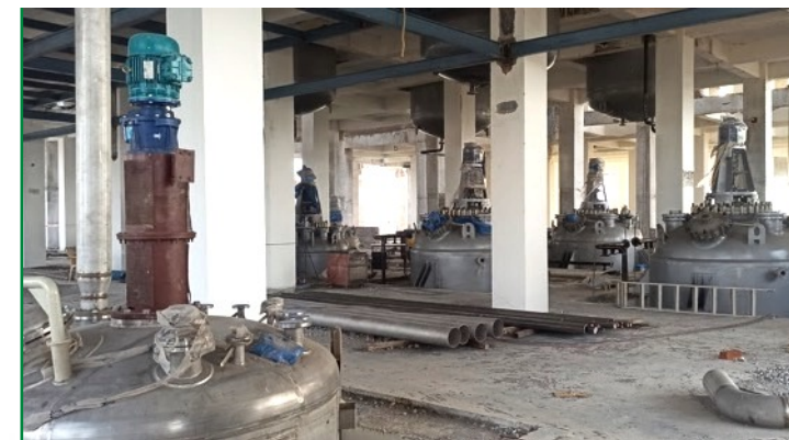
Reactors Installed & Piping Commenced
