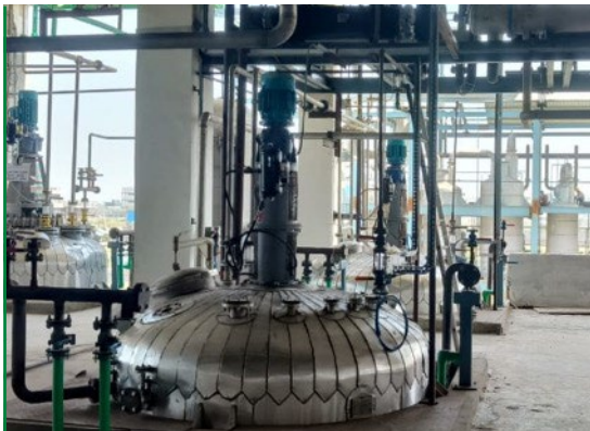
Reactor Installation Completed
